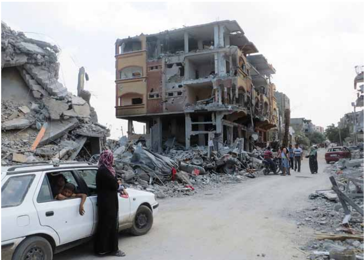
Damage to homes in Beit Hanoun.
